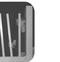
**Step 11:** Starting at one end, begin inserting spindles into holes in bottom rail.
