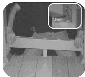
**Step 7:** Slide bracket covers onto both ends of bottom rail. Place bottom rail onto bracket plates making sure rail rests firmly on the two tabs that protrude from the bottom of the bracket base plate.
