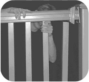
**Step 12:** With bracket covers on rail and spindles installed in bottom rail, place top rail into position by feeding rail down onto spindles.
