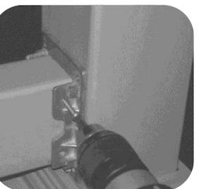
**Step 8:** Pre-drill and secure rail to brackets using (4) 1" stainless steel screws(provided) per bracket. **Important:** Skipping this step will void warranty. Slide bracket covers onto the bracket base plate and press firmly into place. Tap with rubber mallet.
