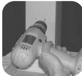
**Step 4:** Pre-drill marked holes for easier application using 1/8" drill bit.
