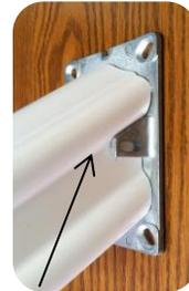
Upper rail section must rest on "down" stair bracket as shown for bracket cover to fit properly.
