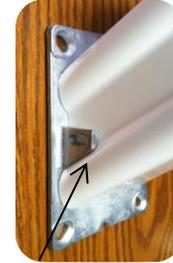
Lower rail section must rest on "up" stair bracket as shown for bracket cover to fit properly.
