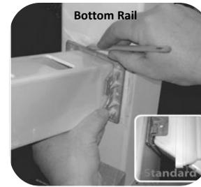
**Step 6:** Keeping bottom rail as close to stair treads as possible, and maintaining desired angle, slide each bracket into position, with Z-Wedge if needed. Rail should rest on lower lip of base plate. Mark the position of the base plate or Z-Wedge on post and remove bottom rail.
