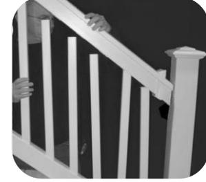
**Step 11:** With spindles installed in bottom rail, place top rail into position by feeding rail down onto spindles. Trustin rail shown in image.
