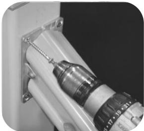
**Step 12:** With top rail resting on spindles, raise top rail 1/4", or to desired height, allowing the spindles to float. Check local building codes for correct stair rail height requirements. Secure mounting plate to post using (4) 2" stainless screws(provided). If Z-Wedge being used, place in-between bracket and post before securing with screws.
