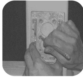
**Step 3:** Place bottom edge of bracket base plate on line marked earlier. Center on post, using as a template, mark the 6 inside screw holes onto the post.
