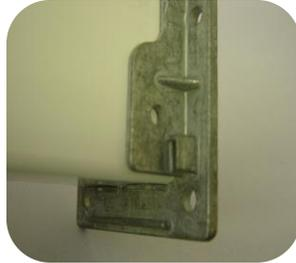
**Step 13:** With top rail properly seated in bracket base plate, pre-drill and secure rail to brackets using (4) 1" stainless steel screws (provided) per bracket. Slide bracket covers onto to bracket base plates and press firmly into place. Tap with rubber mallet.
