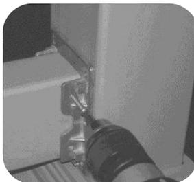
**Step 8:** Pre-drill and secure rail to brackets using (4) 1" stainless steel screws(provided) per bracket. **Important:** Skipping this step will void warranty. Slide bracket covers onto to bracket base plates and press firmly into place. Tap with rubber mallet.
