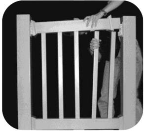
**Step 12:** Slide bracket covers onto both ends of top rail and begin feeding the rail down onto the pickets. Make sure rail is resting firmly on tabs see step 13.
