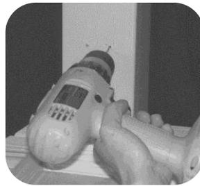
**Step 4:** Pre-drill marked holes for easier application using 1/8" drill bit.
