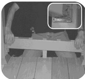
**Step 7:** Slide bracket covers onto both ends of bottom rail. Place bottom rail onto bracket plates making sure rail rests firmly on the two tabs that protrude from the bottom of the bracket base plate.
