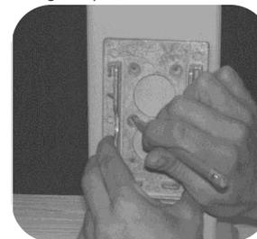
**Step 10:** Place bottom edge of top rail bracket base plate on line marked in step 9. Center on post, using as a template, mark the 6 inside screw holes onto the post. Use 6 outside holes for adjustable post mount. Repeat steps 4 and 5 for top bracket.
