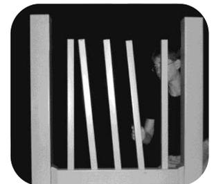
**Step 11:** Starting at one end, begin inserting spindles into holes in bottom rail.
