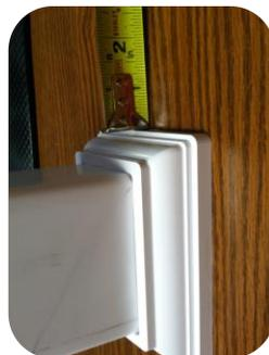
**Step 9: Top rail bracket placement:** With bottom rail bracket cover installed, measure from top of bottom rail bracket cover and make a mark on post. 36" tall rail kit, mark at 25 11/16" 42" tall rail kit, mark at 31 11/16"
