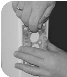
Bottom Rail Bracket Attachment
