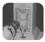
Step 5: Attach bottom bracket base plate to post using (6) 2" stainless steel screws(provided) per bracket. Bracket tabs need to be towards bottom of base plate when installed.
