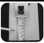
**Bottom Bracket Placement:** Before sleeving posts, mark bottom bracket position by measuring from bottom of post sleeve.
