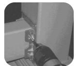
Step 8: Pre-drill and secure rail to brackets using (4) 1" stainless steel screws(provided) per bracket.
