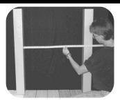
**Step 1:** Slide on post sleeves. Measure distance between sleeved posts, if needed; make any adjustments to rail length. See cutting notes. If installing custom pre-assembled railing sections, no adjustments are necessary.
