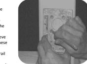
**Step 10:** Place bottom edge of top rail bracket base plate on line marked in step 9. Center on post, using as a template, mark the 6 inside screw holes onto the post. Use 6 outside holes for adjustable post mount. Repeat steps 4 and 5 for top bracket.
