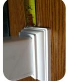
Step 9: Top rail bracket placement: With bottom rail bracket cover installed, measure from top of bottom rail bracket cover and make a mark on post.
