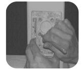
**Step 3:** Place bottom edge of bracket base plate on line marked earlier. Center on post, using as a template, mark the 6 inside screw holes onto the post.
