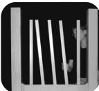
**Step 11:** Starting at one end, begin inserting spindles into holes in bottom rail.
