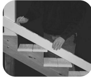
**Step 1:** Lay the bottom rail as close to the treads as possible and up against the posts. While maintaining either a 34° or 39° downward angle. Keep the spacing between the first spindle hole and post equal on either end. Clamp rail to post.
