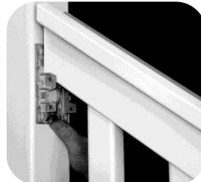
**Step 12:** With top rail resting on spindles, slide the bracket base plate into position; with Z-Wedge if needed, making sure the rail is seated in bracket correctly. Raise rail 1/4" from resting position or to desired height, allowing spindles to float. Check local building codes for correct stair rail height requirements. Mark bracket location on post. Repeat for other bracket. Remove rail and repeat Step 7.
