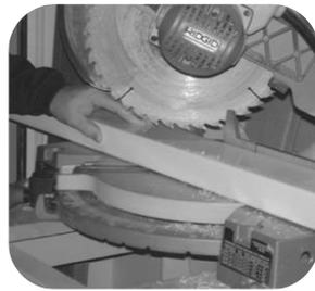
**Step 4:** If Z-Wedge is not required; subtract 1/8" per side (1/4" total) to allow space for the bracket base plates. Miter cut both the top and bottom rails, including aluminum reinforcement.
