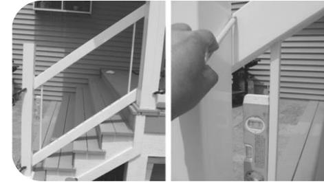
**Step 2:** Place a spindle in the first and last spindle hole, set top rail and plumb spindles. Clamp top rail to post, using a pencil, draw miter lines on top and bottom rail.
