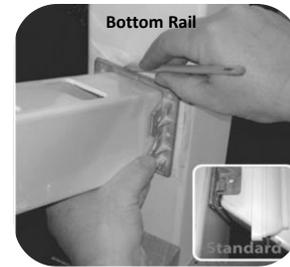
**Step 6:** Keeping bottom rail as close to stair treads as possible, and maintaining desired angle, slide each bracket into position, with Z-Wedge if needed. Rail should rest on lower lip of base plate. Mark the position of the base plate or Z-Wedge on post and remove bottom rail.
