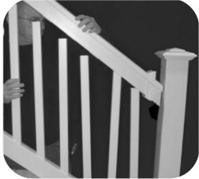
**Step 11:** With spindles installed in bottom rail, place top rail into position by feeding rail down onto spindles.
