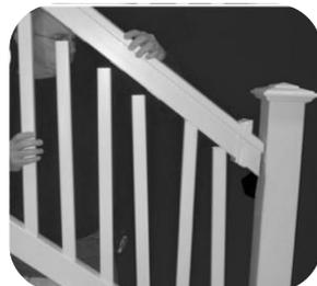
**Step 13:** Slide bracket covers onto both ends of top rail. Remember, lower rail bracket cover is taller than upper rail bracket cover. Place top rail into position by feeding rail down onto spindles and resting rail into installed bracket base plates. Pre-drill and secure rail to each base plate using (4) 1" stainless steel screws. See step 8.
