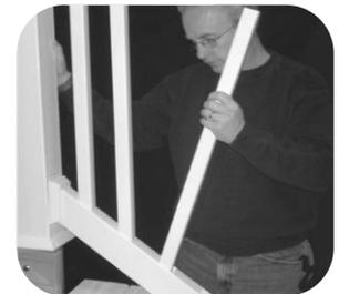
**Step 9:** Starting at one end, begin inserting spindles into holes in bottom rail
