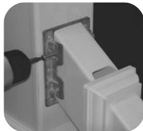
**Step 7: NO Z-Wedge:** Using the base plate as a template mark locations of the 6 **inside** holes and pre-drill with 1/8" bit. Use 6 outer holes for adjustable post mount. Attach both base plates using 6-2" stainless steel screws(provided) per bracket. Lip must be at bottom of base plate.
