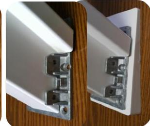
Lower rail section must rest on stair bracket as shown for bracket cover to fit properly.
